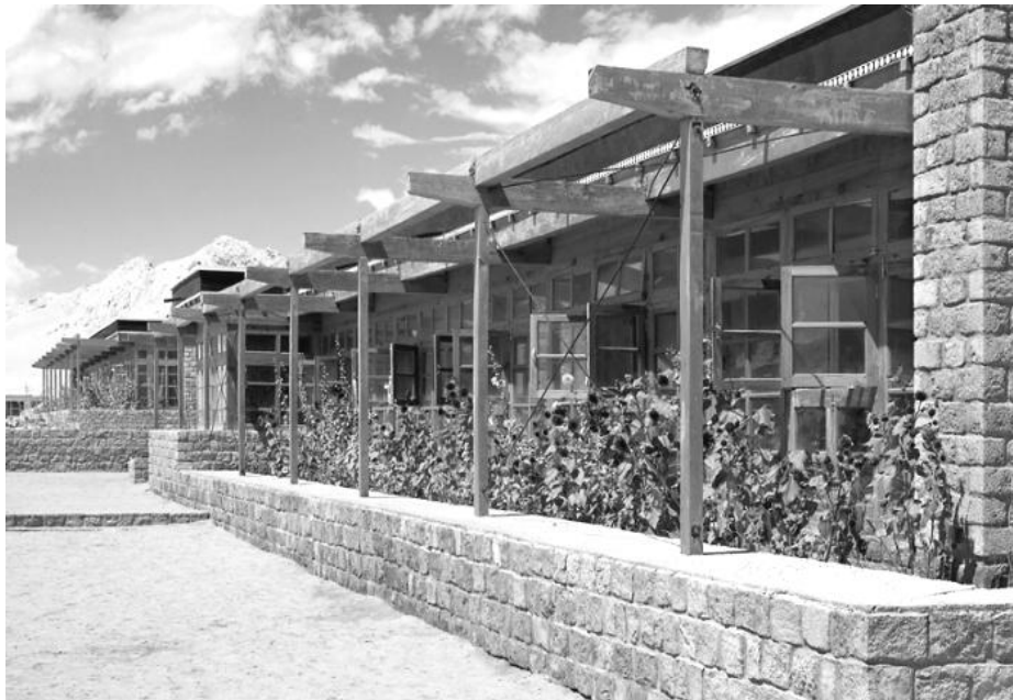
Fig. 3: Energy efficient Trombe walls at Druk white lotus school, Ladakh, India [9]
